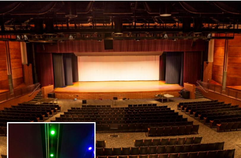
Illuminated Integration installed a complete LED theatrical lighting system for Oxford Area High School's Auditorium. The existing incandescent ellipsoidal fixtures were retrofitted with new LED sources. New color changing wash fixtures were installed over the stage. The ETC control system was upgraded to provide simple control and advanced control from both wall mounted touchscreens and a theatrical lighting console.
