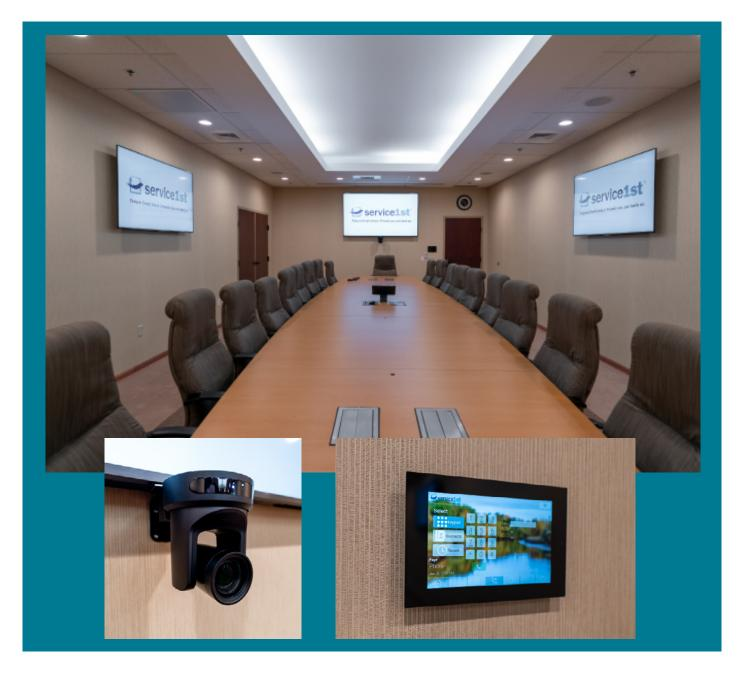
Illuminated Integration installed a audio and conference video system in Service First's Corporate Conference Room. Our Integrations Team set up a system controlled by a mounted touchscreen, or portable iPad to control the conferencing camera, televisions, phone system, and audio capabilities.
